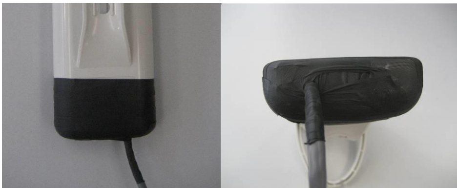
Figure 2-8 First Layer-Rubber Tape
