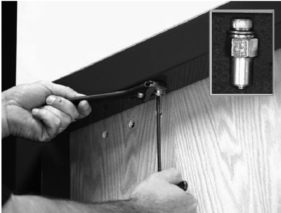
Figure 9. Installing the Blind Nuts
