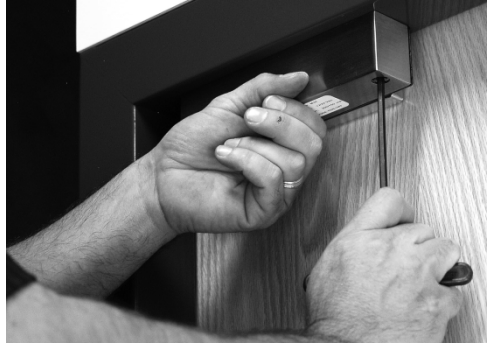
Figure 17. Installing the Magnalock
