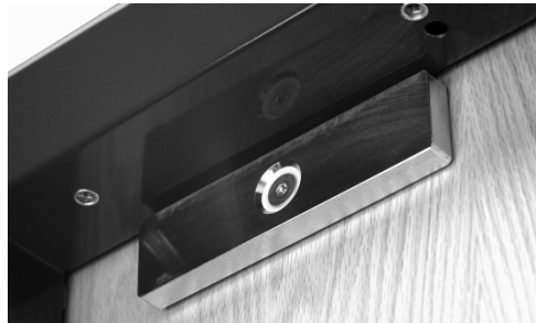
Figure 16. Installing the Strike Plate
