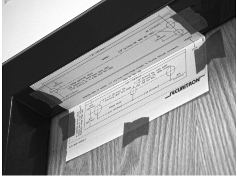
Figure 4. Attaching the Template
