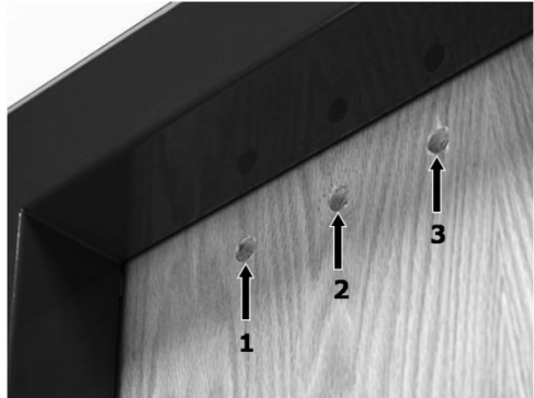
Figure 6. Installation Drill Holes
